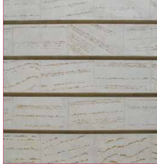
Fig. 5 - Decorative concrete finishing detail (photo Alvisi 2014).
