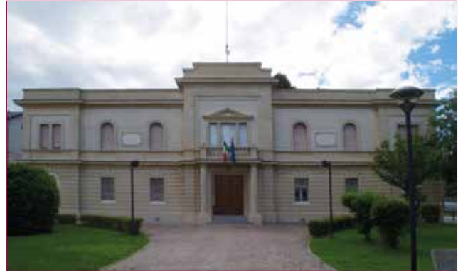
Fig. 11 - The main front of Camposanto city hall after the restoration works (photo Alvisi 2016).
